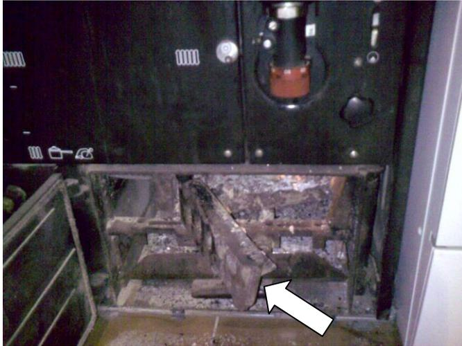
To light a fire please open the lid of the fire room on top of the oven. Pile up in the front corner approx. 10 pieces of kindling wood in form of a pyramid and set a nest of paper below. Then open the tin door in the front of the oven pull the locking handle of the door into the upright position and open first this door and then behind the door the shutter to the fire room (see arrow).
