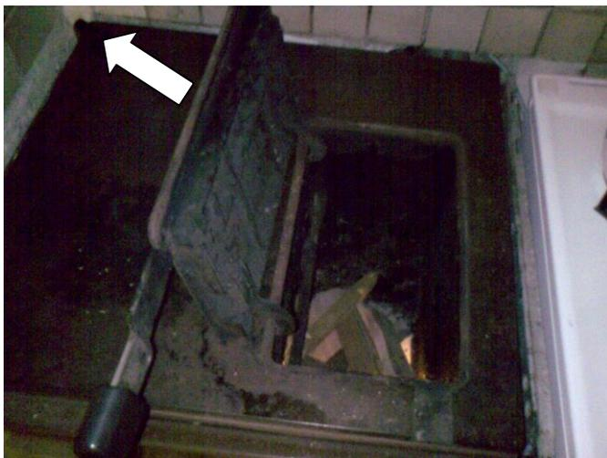
The central heating and the additional hot water is heated by the wood oven in the kitchen. To start the fire first make sure that the air lid on the left hand upper corner of the hearth is fully opened, i. e. turn it fully to the right position. As long as a fire is burning in the oven the lid must not be closed. Whenever the lid is closed while fire is burning there is the risk of a flash fire or smoke may fill the kitchen. Instruct all persons accompanying you!
